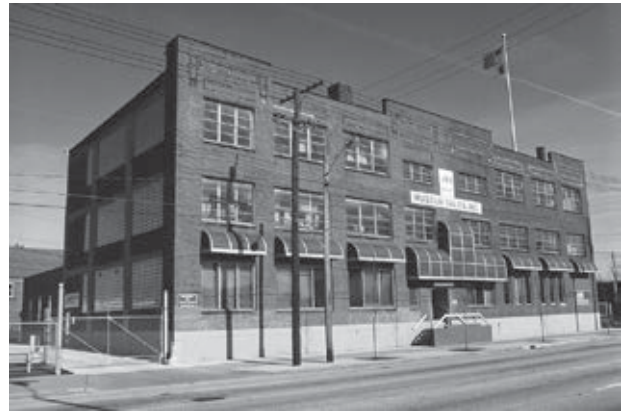
Cleveland Sales Office, Warehouse, and Learning Center
