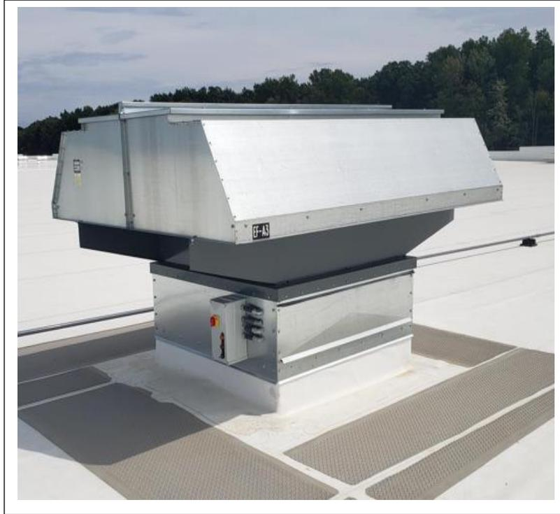
Cook now offers an integral starter solution which eliminates the messes of multiple wall mounted starters and extensive wiring with long runs.
